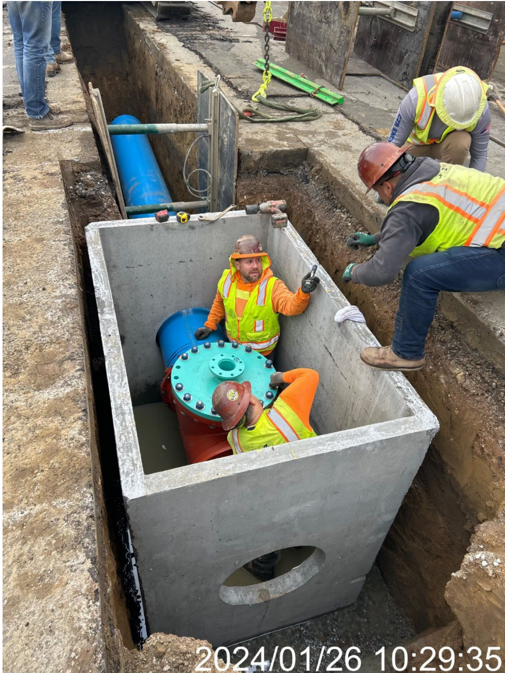
Installing precast vault and valve, January 26, 2024, Old County Road
