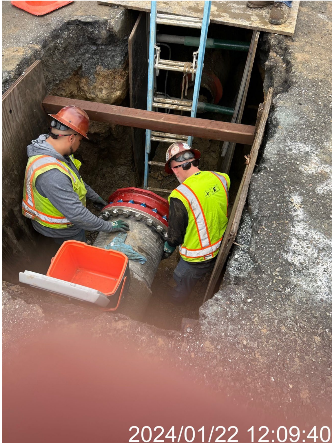
Flange install on 20-inch line, January 22, 2024, Old County Road
