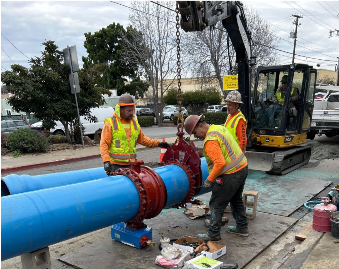
Installing 20-inch pipe, January 26, 2024, Old County Road
